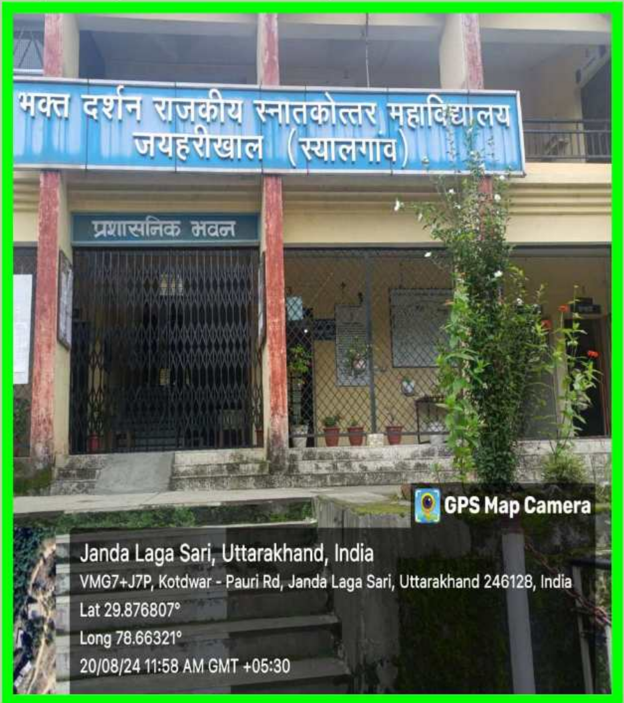
Ramp at College administrative Building
