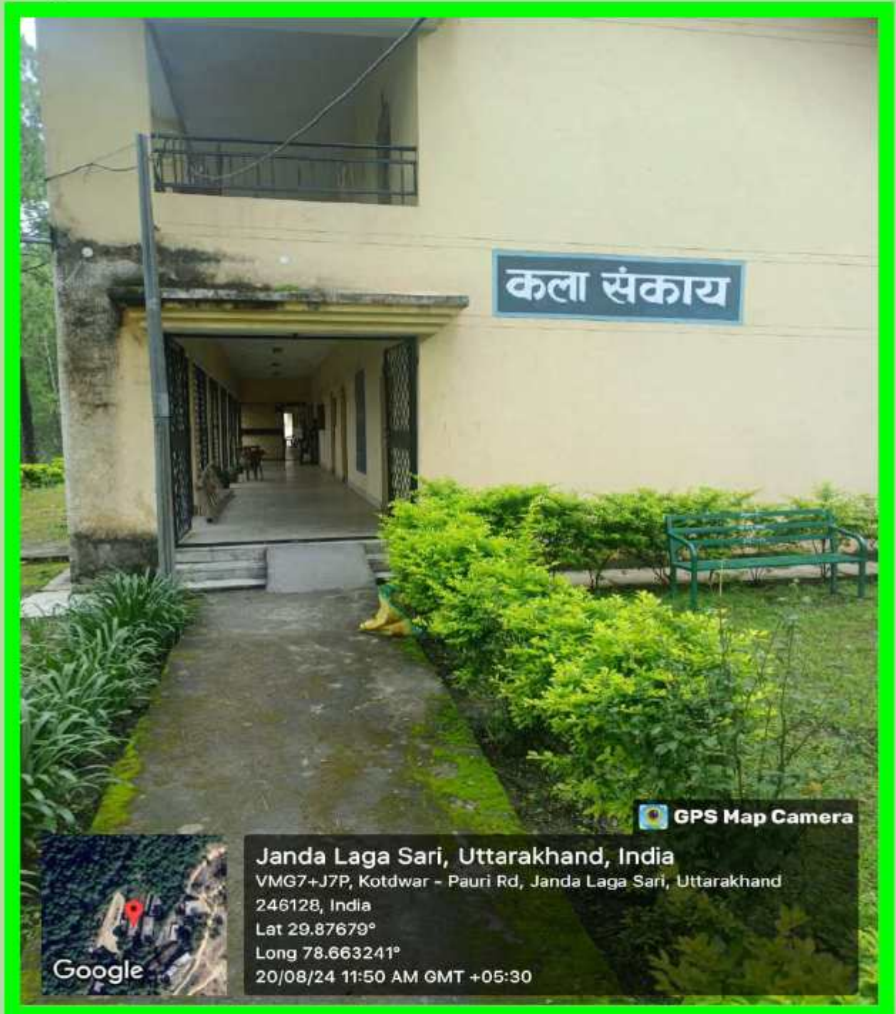
Ramp at Arts Block
